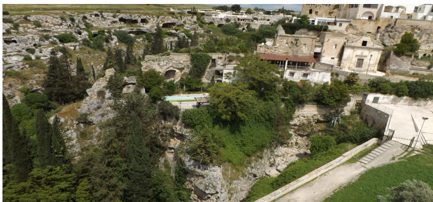
Figure 2. Rupestrian Complex located in front of the historic centre, on the other side of the crevasse.
